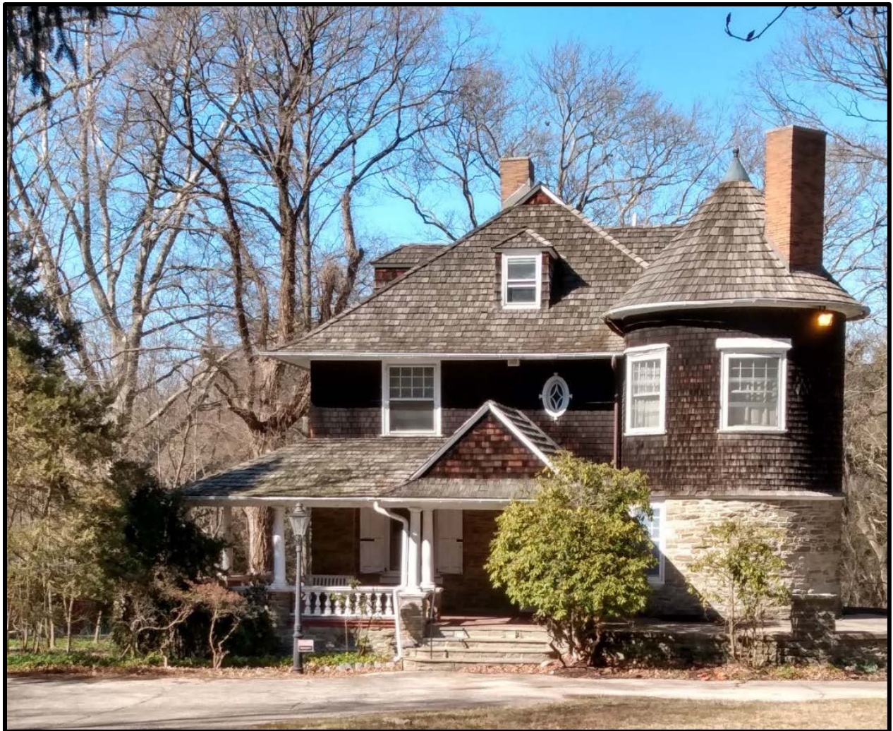
Figure 6 Front of the house (south façade, looking north)
