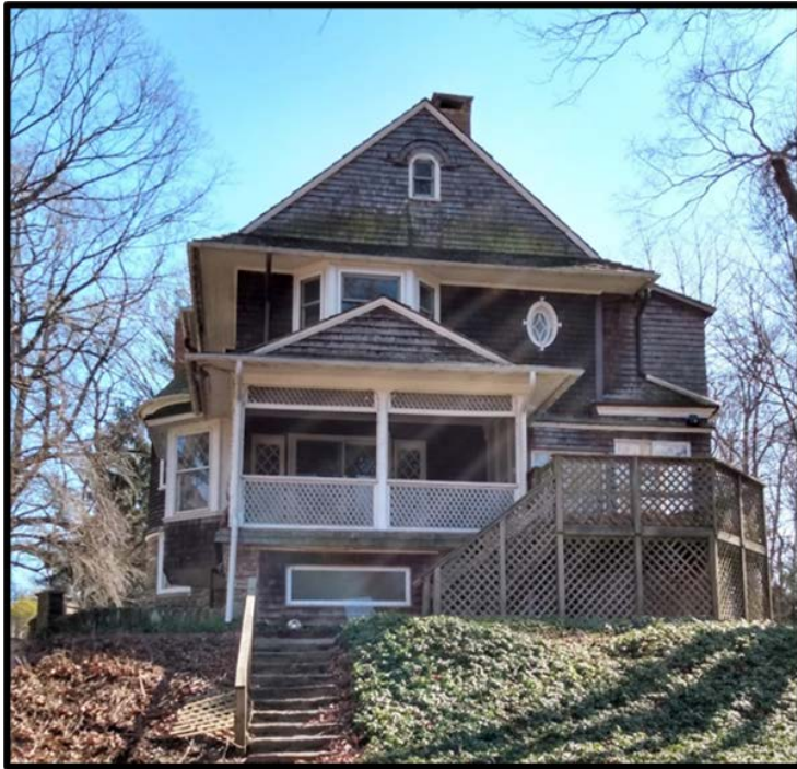
Figure 12. Rear of house
