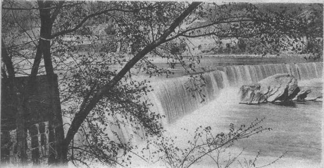
349. PHILADELPHIA— FLAT ROCK DAM, SHAWMONT
