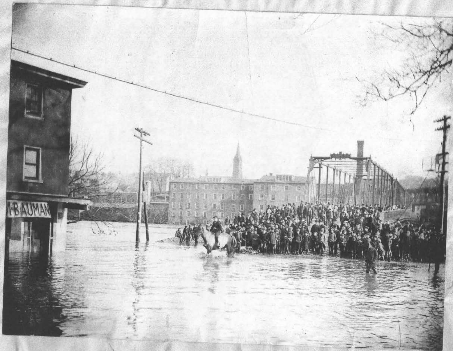
West Manayunk. Aftermath of the flood of February 28th 1902, at the old Pay Bridge, at Green lane. Picture taken from west end of structure, on morning of March 1st, 1902, when the water had lowered three feet.
