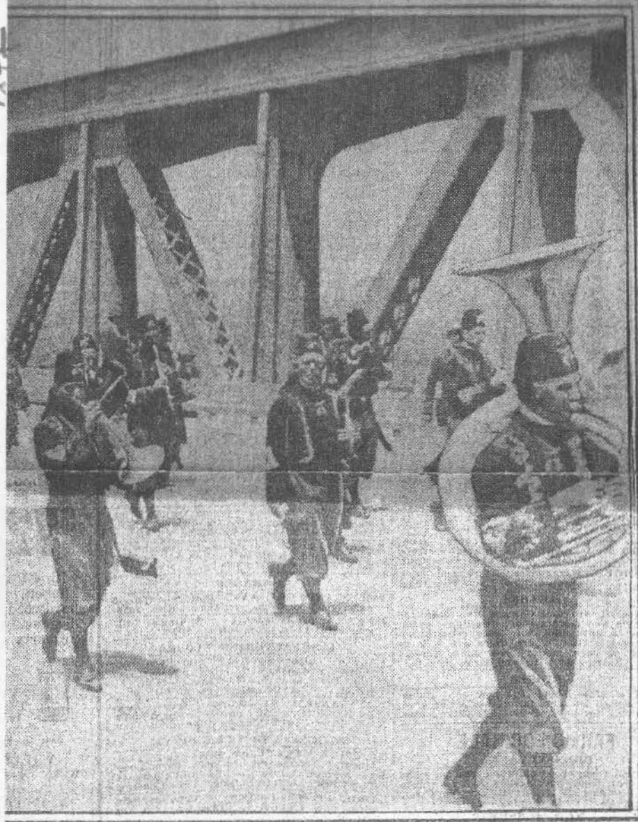
PROCESSION OF THE DELAWARE RIVER BRIDGE yesterday led a gay procession across the huge suspension structure between Pennsylvania and New Jersey
