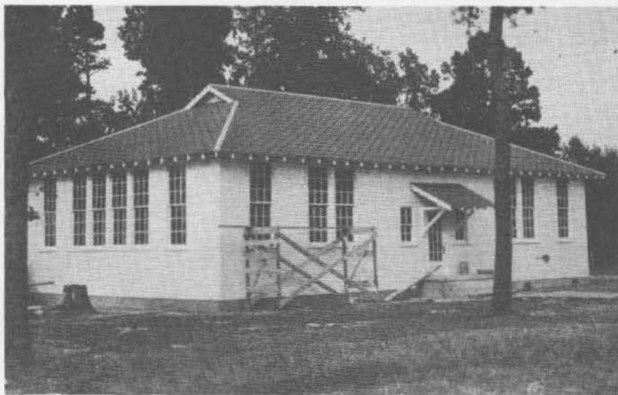
Construction of Star City School at Star City, Lincoln County, Arkansas, by WPA workers.
