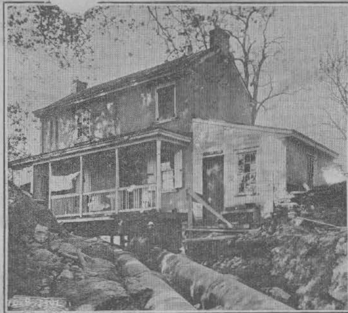
NO COAL, BUT PLENTY OF WATER IN THIS CELLAR.
