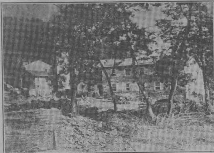
Upper Magarge Paper Mill, at Thomas Mill Road, Wissahickon Creek. The photograph was taken in the early 1870's, a few days after a great freshet had demolished the red, covered, bridge leading to the mill. The picture is reproduced through the kindness and courtesy of a grandson of Charles Magarge.
