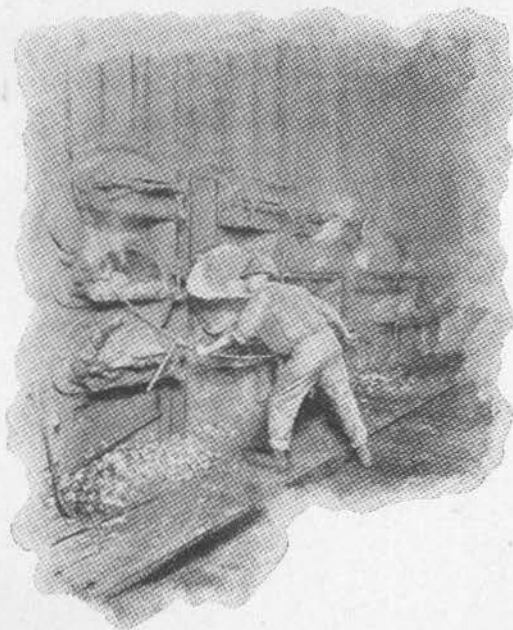
CLEANING STANDPIPE RETORT HOUSE
