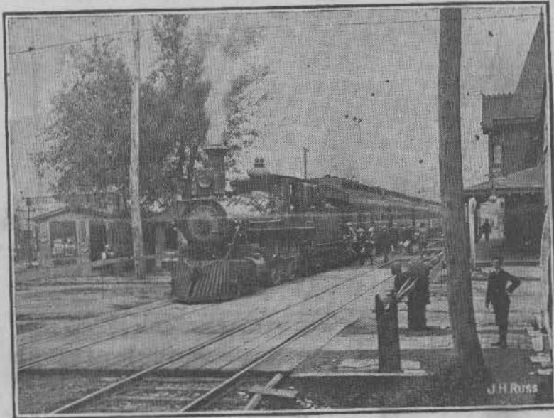
CHELTEN AVENUE GRADE CROSSING WHICH WILL BE ELIMINATED.
