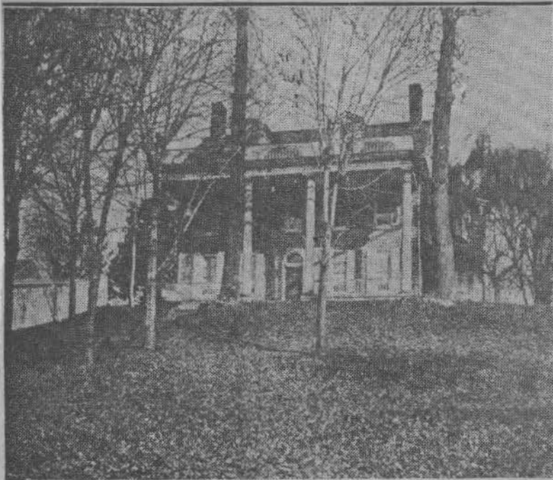
Picturing the old Mansion, at the Falls of Schuylkill, which was built by Thomas Mifflin prior to the Revolutionary War. It was here that Mifflin resided when he served as Chief Executive of Pennsylvania. The structure was located on the hillside, above Ridge avenue, between what is now Stanton street and Midvale avenue. It was torn down in 1893.
